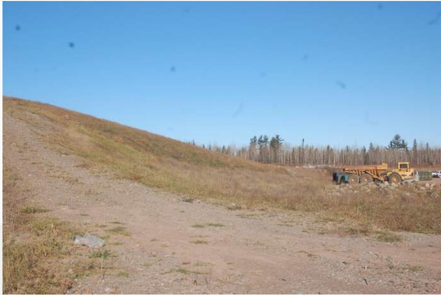
Photo 7 - Phase 1 East Waste Slope
