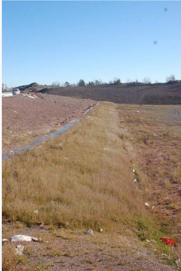
Photo 15 - Phase 3 and 4 South Exterior Slope
