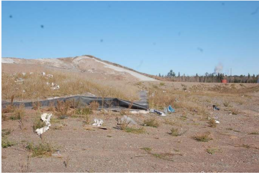
Photo 11 - Phase 3 East Exterior Slope
