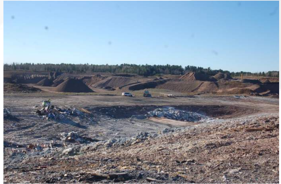
Photo 2 - Phase 3 and 4 Lower Active Area
