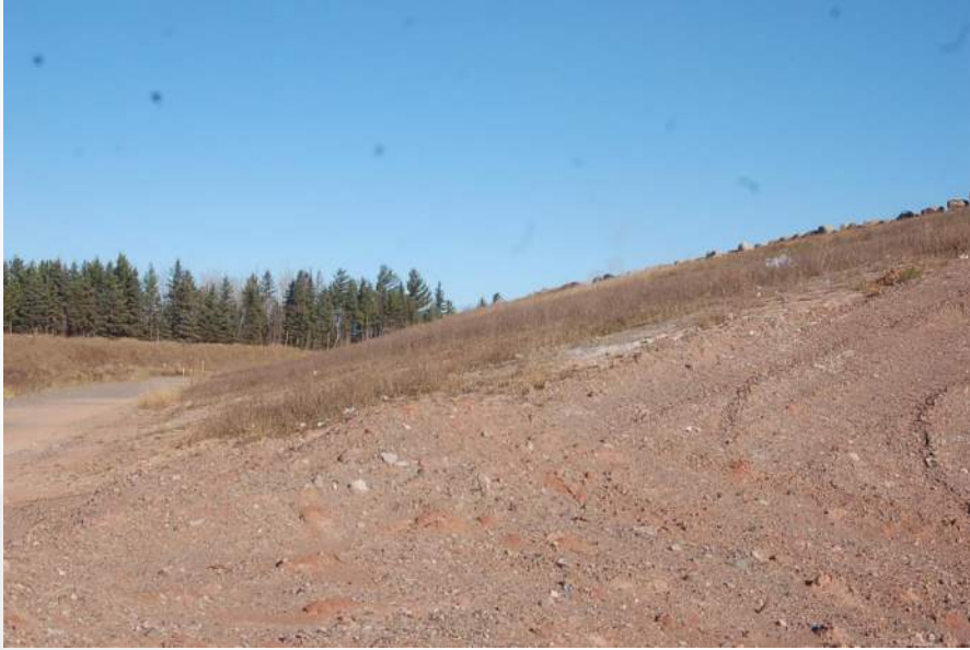
Photo 17 - Phase 2 West Waste Slope
