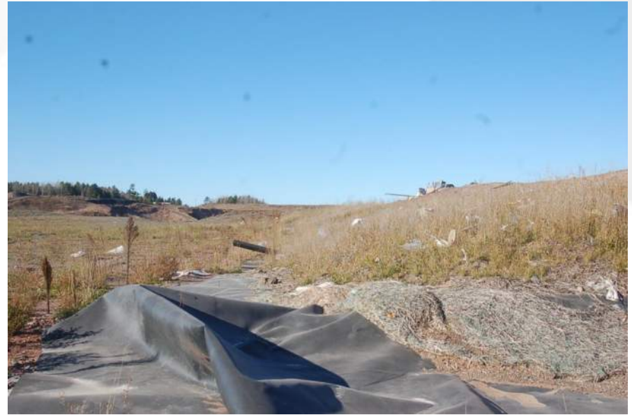
Photo 12 - Phase 3 South Exterior Slope
