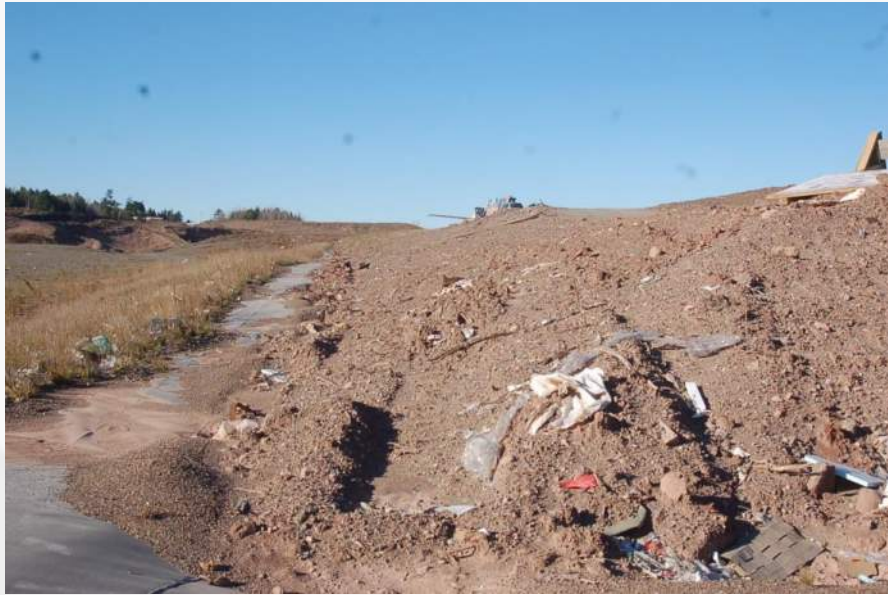
Photo 13 - Phase 3 South Working Face
