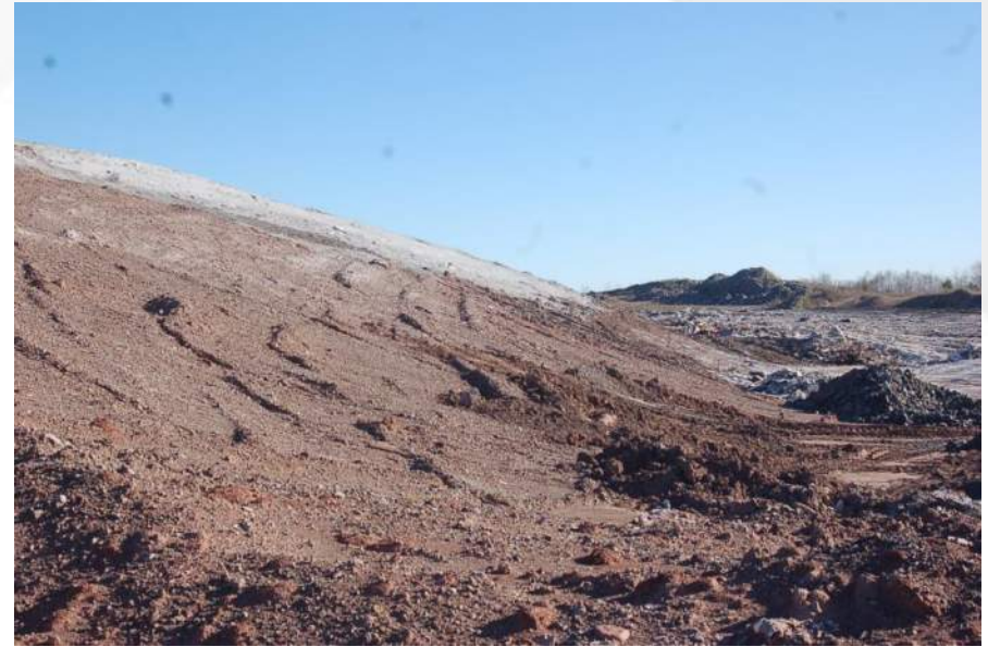
Photo 16 - Phase 1 and 2 South Internal Working Slope
