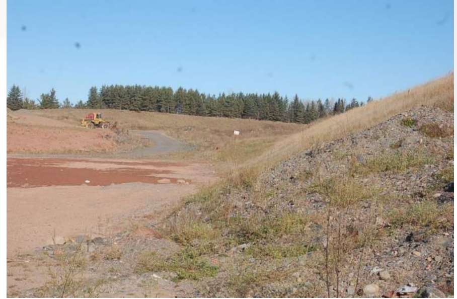
Photo 18 - Phase 2 West Exterior Slope
