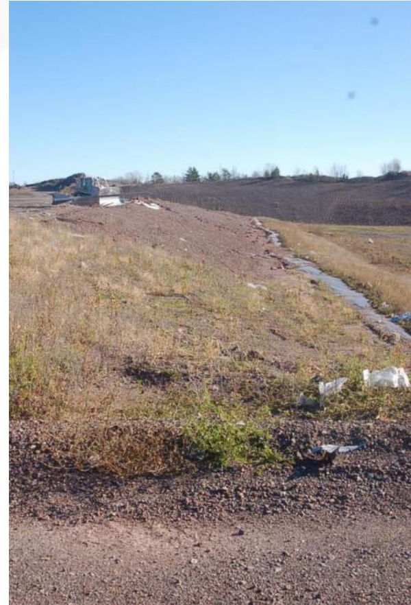
Photo 14 - Phase 3 and 4 South Working Face
